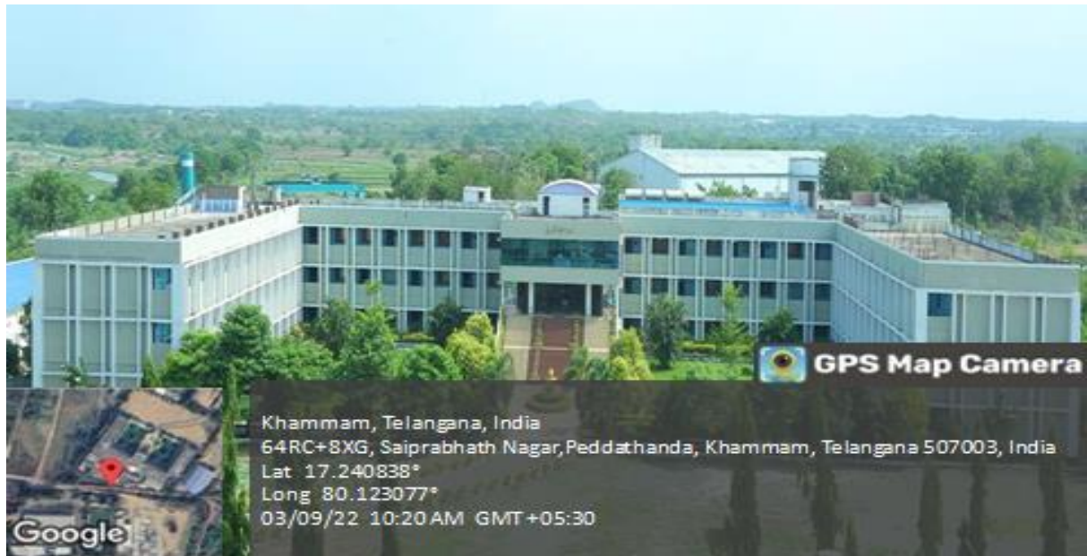
Fig 15: Areal View of college
